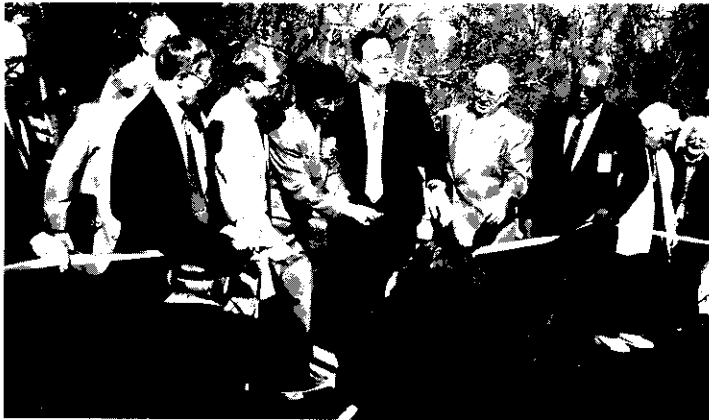
Dedication of the newly restored Abbott Bridge.
