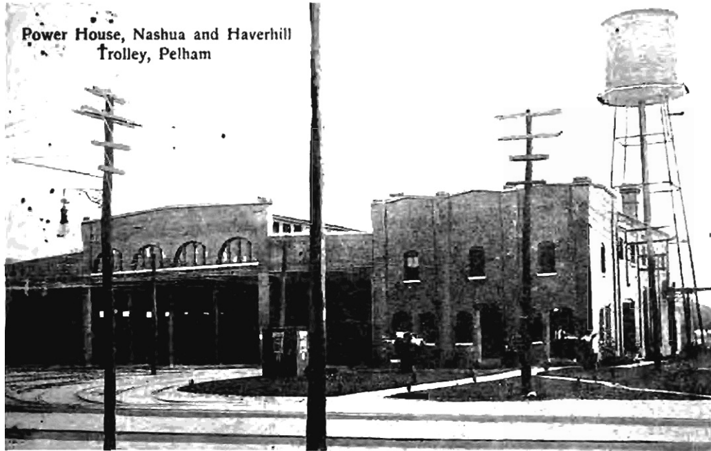
Here's the Pelham carhouse and rotary station in 1903. The large tank supplied water for the building's automatic sprinkler system.
