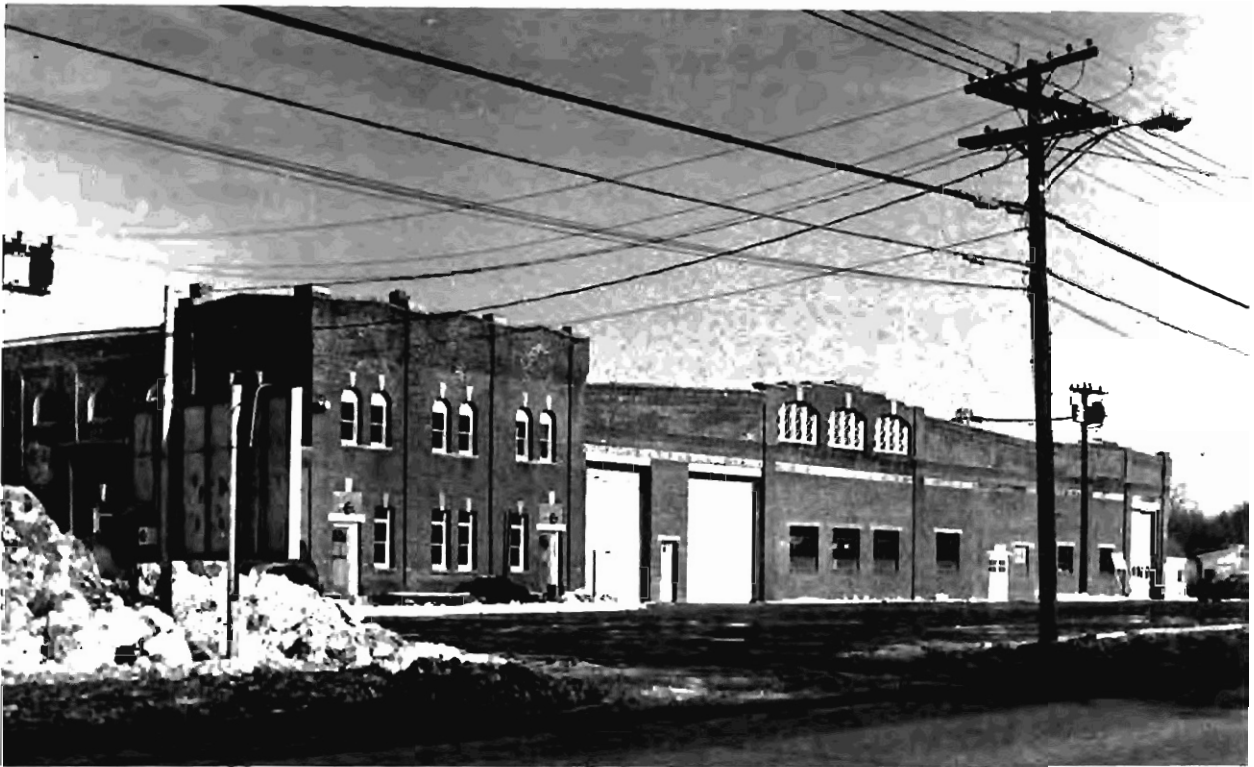
Now housing the Canobie Shoe Company and other industries, the old Salem carhouse is still easily recognizable as a former car barn.
